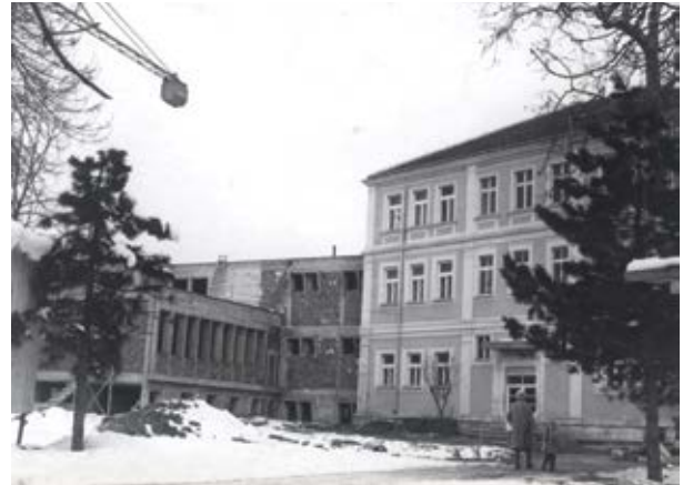
Construction of the new wing of the Library
